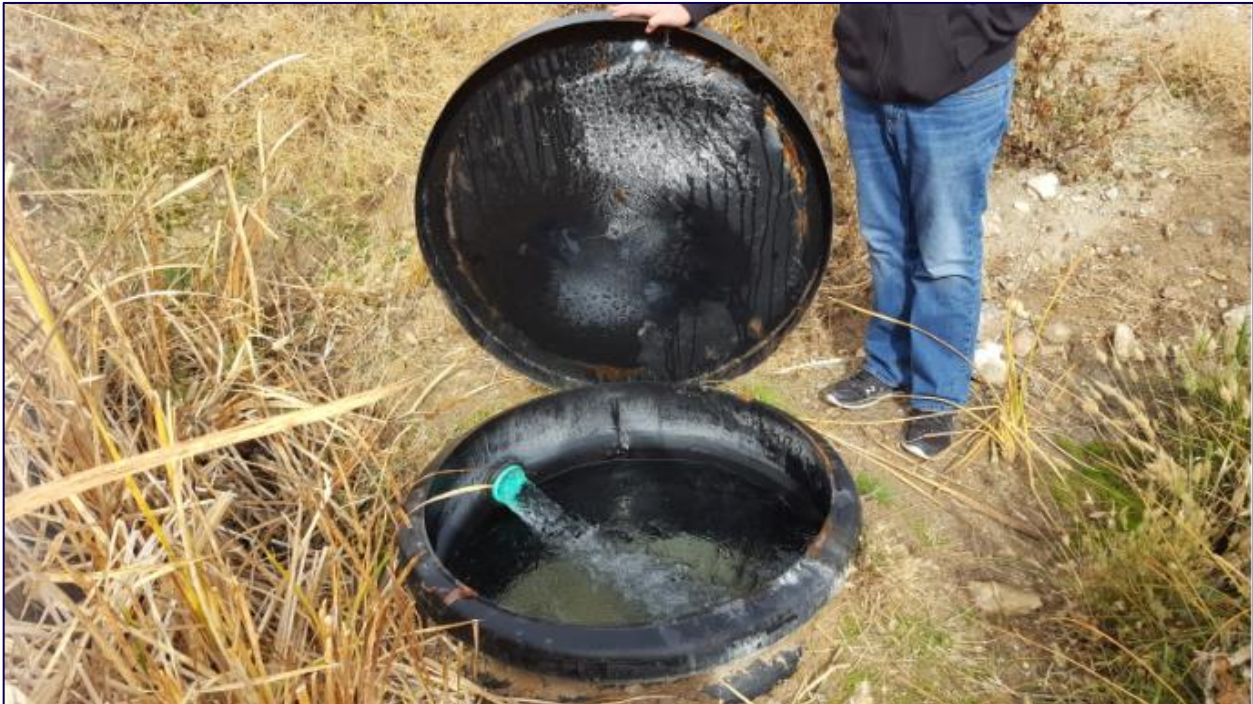
Redlum Spring Wellhead – photo Steve Allison
